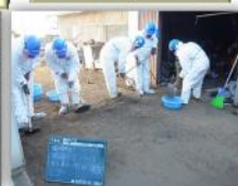
Garden: removal of topsoil
