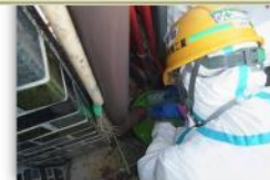
Gutter (vertical): high-pressure water cleaning
