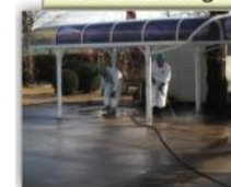
Concrete floor: High-pressure water cleaning
