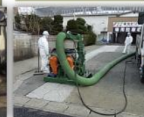
Concrete floor: Shot blast
