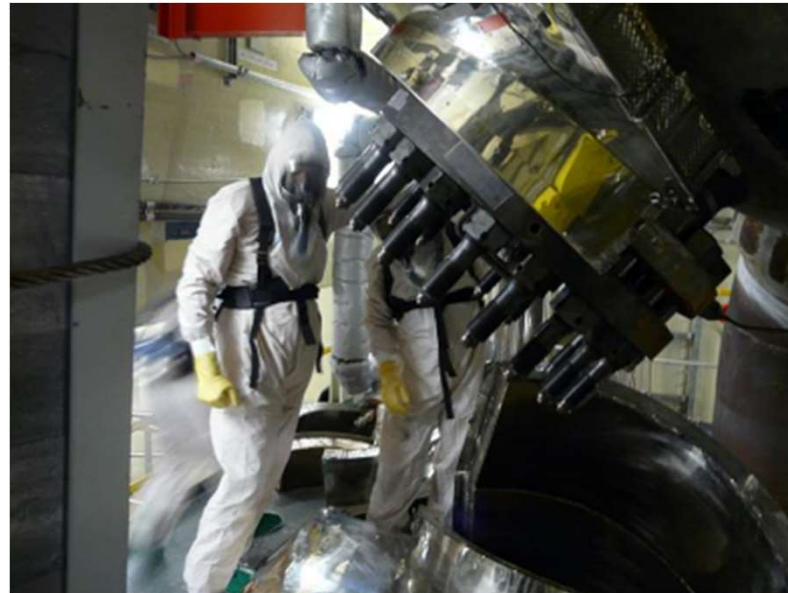
Inspection of a steam generator © EPZ, 2018
