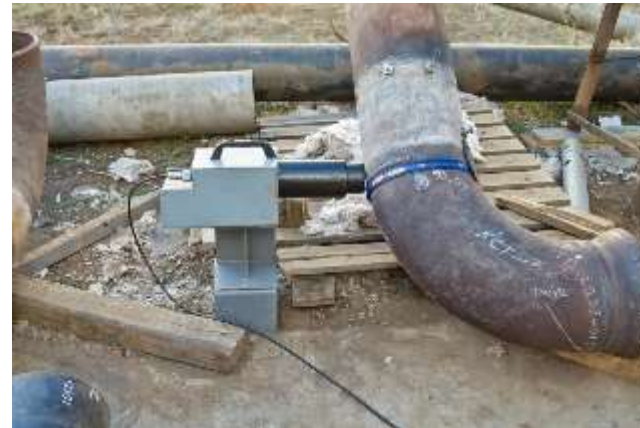
Inspection of welds thick-walled tube © Shinobi /Shutterstock.com, 2018.
