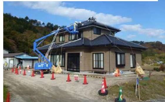
Washing and brushing of roofs and walls with pressured water, sanding...
