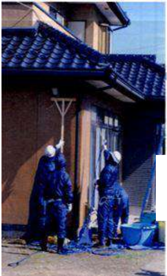
Washing and brushing of roofs and walls with pressured water, sanding...
