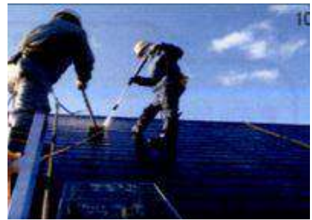
Washing and brushing of roofs and walls with pressured water, sanding...
