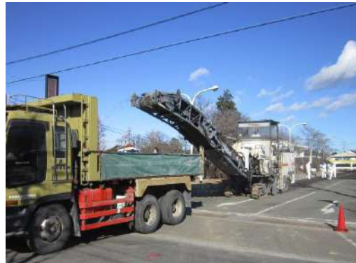
Asphalt removing
